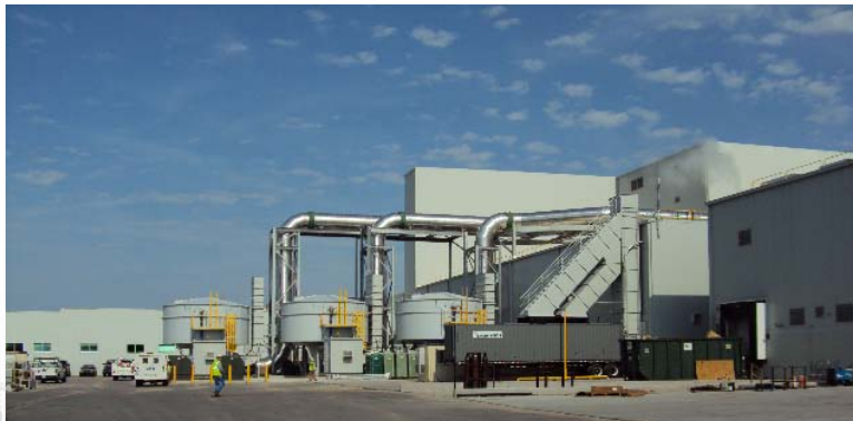
Photo left: Regenerative thermal oxidizers
