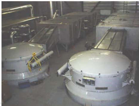
Photo left: Air treatment unit incl. bag filter
