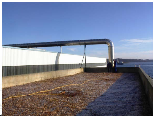
Photo left: Bio filter with wood chips
