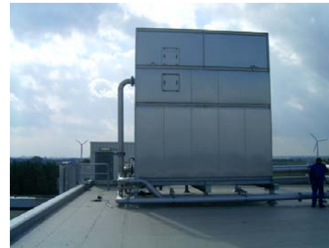
Photo left: Air treatment unit incl. bag filter
